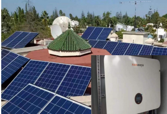
Turkey 220kW Commercial Project
